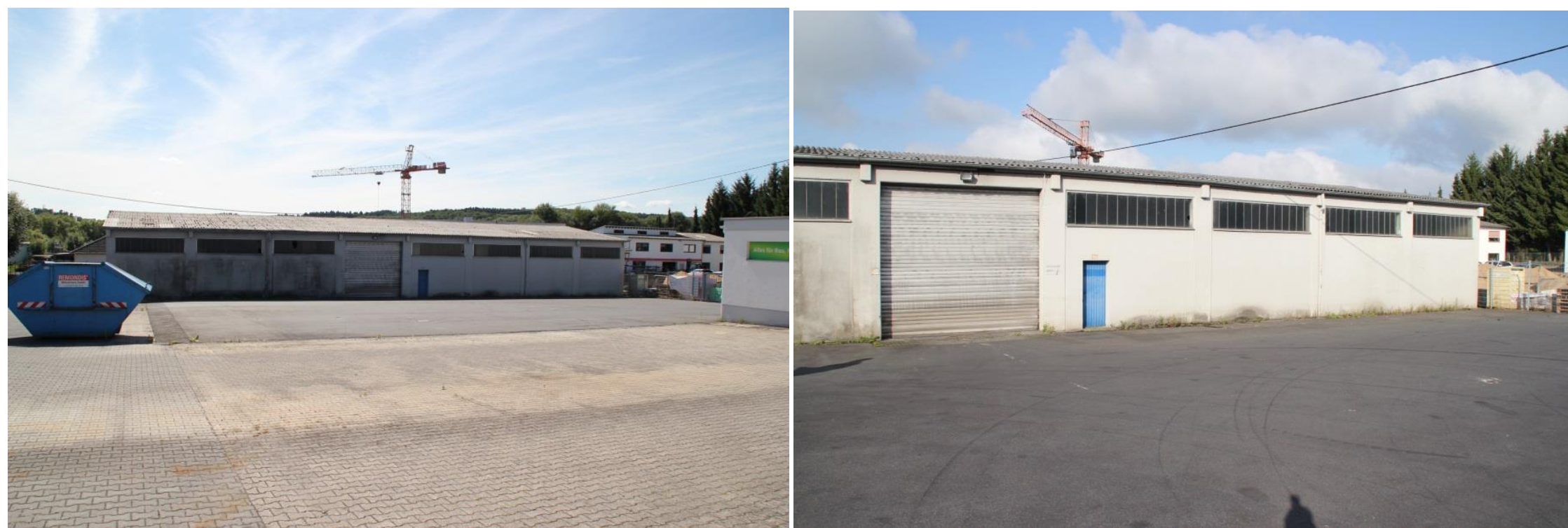
Offene Lagerhalle 22,75m x 7,20m (ca. 180m 2 )
